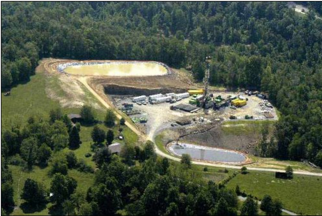
Well pads and brine pits
