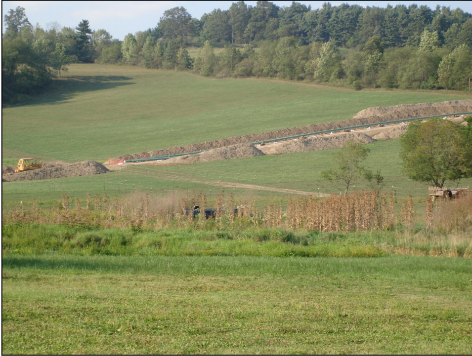
Pipeline Construction (photo Carol Chock)
